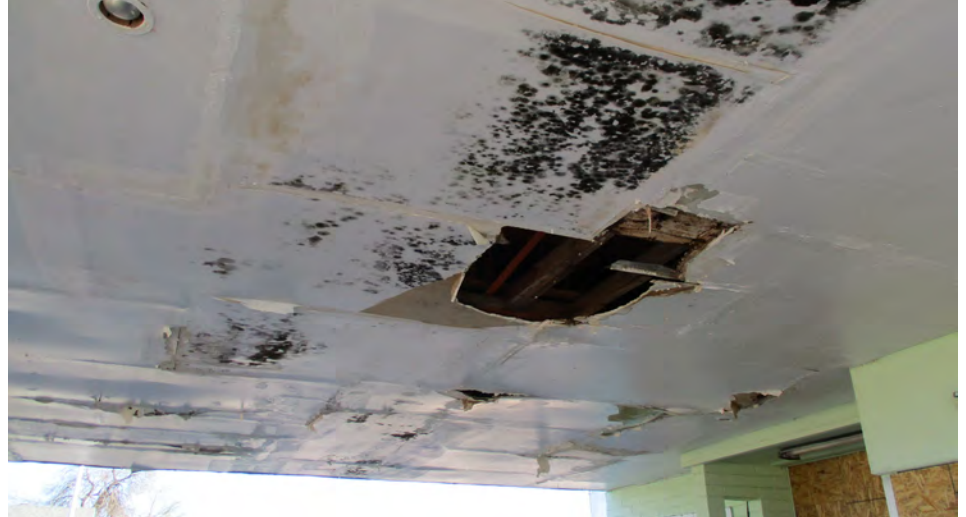
Ceiling at porte-cochere
